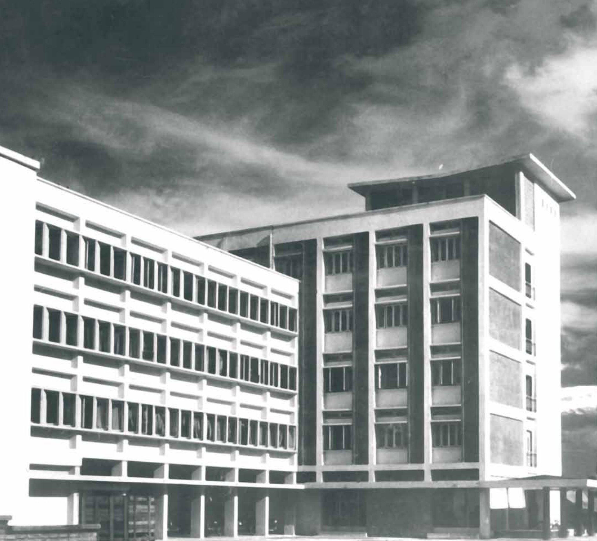
The erstwhile ESIC Headquarters Building
